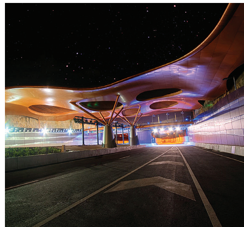
Clem Jones Tunnel — Brisbane
